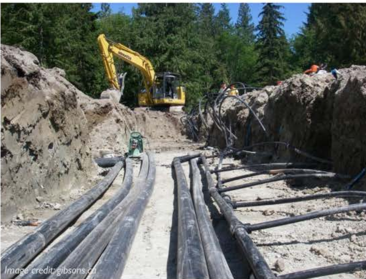
Laying the pipes in the ground
