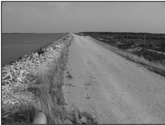
A stretch of the dyke near the highway.
