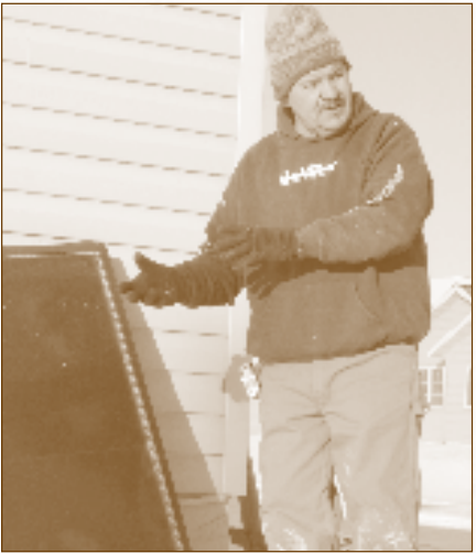
Henry Red Cloud of Lakota Solar Enterprises trains youth in solar heating panel installation.
