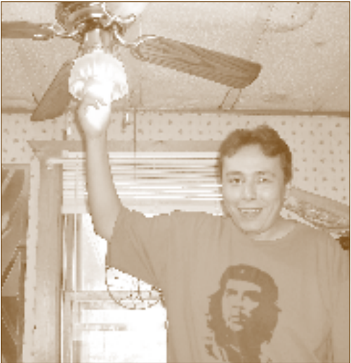
John Shimek installs an energy-saving compact florescent light bulb in a White Earth home. Photo courtesy of WELRP.
