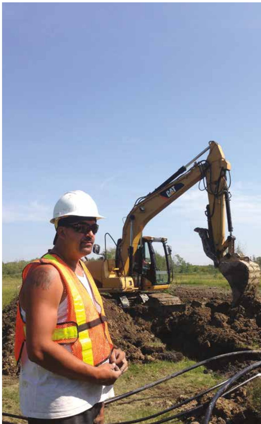
FISHER RIVER BUILDERS INSTALLING GROUND LOOPS FOR GEOTHERMAL HEATING SYSTEMS.
