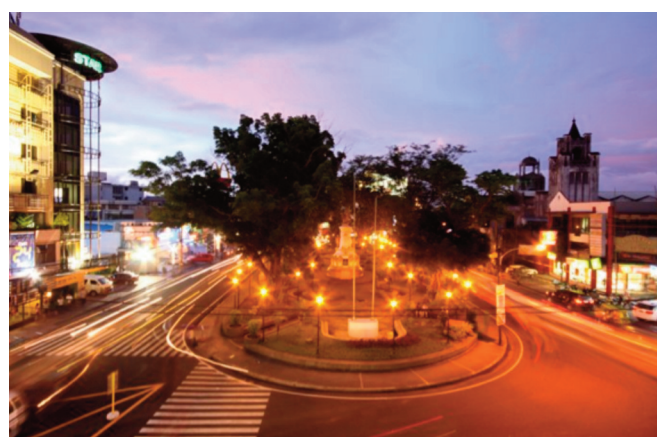
Part of the Central Business District (CBD). More popularly called by locals as "centro", CBD-I is the traditional commercial hub. The Naga River, Hernandez Avenue and Arana Street bound this 30-hectare area. Being the location of most businesses engaged in services and wholesale and retail trade, CBD-I teems with people — which swells to as much as 250,000 during the daytime — from the city and its neighboring municipalities. The Naga City Supermarket, the biggest in Southeast Asia when it was built in 1969, is found at the core of this district.
