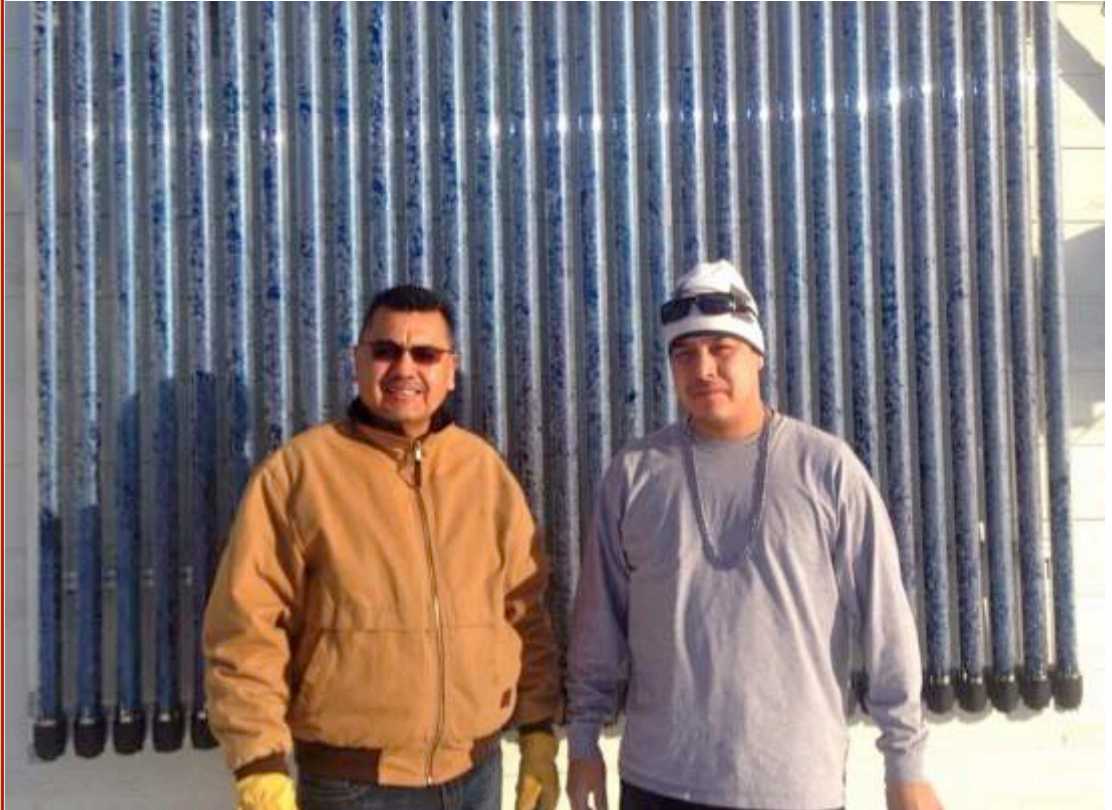
Solar Thermal Hot Water Heating Systems installed by Chief Peguis Construction in 2014.
